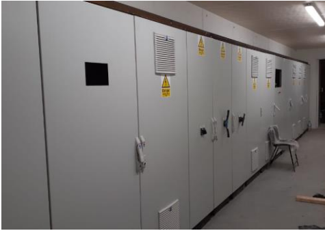
21 T/PH Dry Recycling Plant in Swindon, UK
